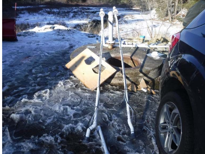
Figure 4: Nozzle piping being routed from vault 1-24-17
