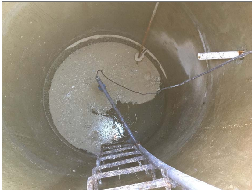
Figure 9: Trial Day 33 (Last Day of Trial) FOG buildup results (2-27-17)
