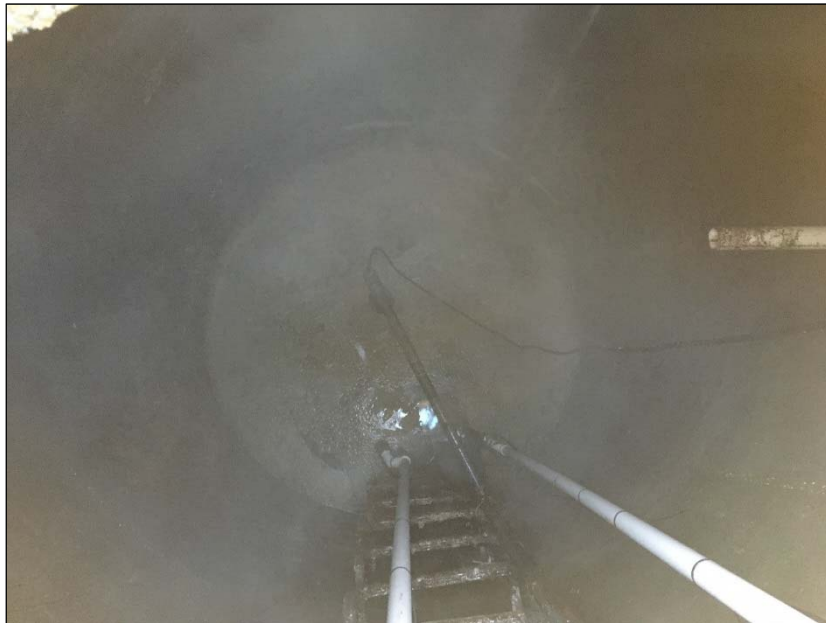
Figure 7: Trial Day 5 – FOG buildup results – 1-30-17
