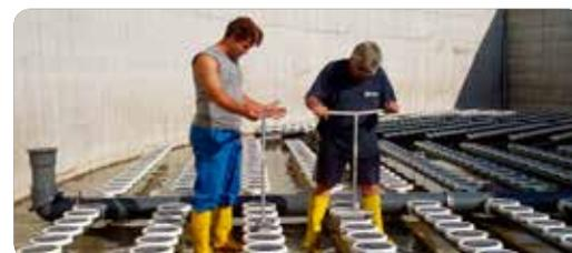
Sanitaire diffusers are designed to provide efficient and reliable biological treatment of wastewater. However, fouling and scaling have a significant negative effect on diffuser performance over time, which result in less effective treatment and rising energy costs.
